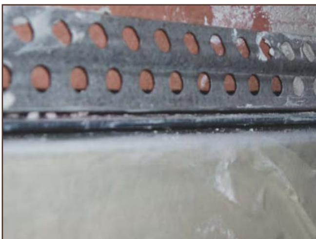
Keep the angle beads at a distance with 2 mm spacers.
