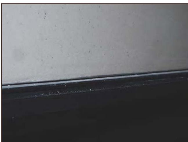
Then Plaster the wall, and make the clearance clean and free from plaster residue.
