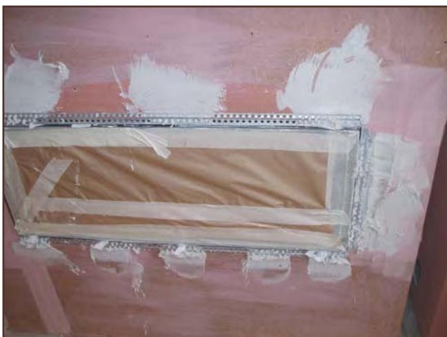
Then attach the angle beads around the recess frame at 2 mm distance from the recess frame.
